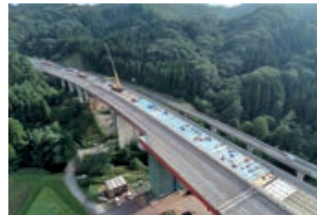
Example of bridge deck slab replacement work
