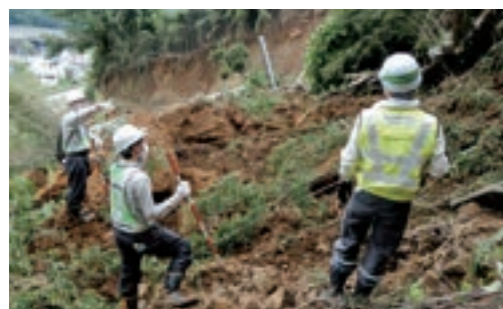
Onsite restoration support by expert technicians
