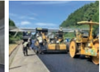
Pavement repair work
