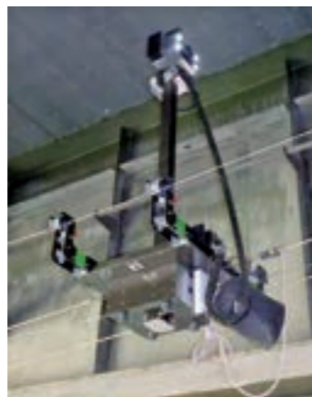
Inspection of the underside of the viaduct deck slab
