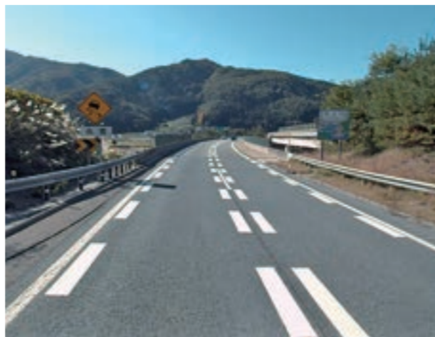
Leading lane marks (Broken lines)
