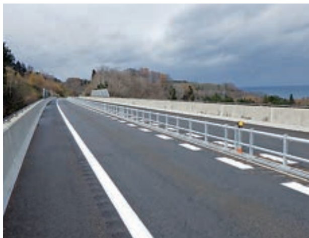
Center pipe divider at the viaduct section
