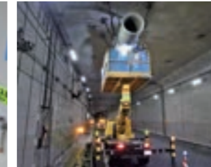
Cleaning of tunnel ventilation equipment
