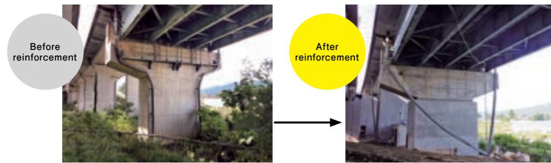
Seismic reinforcement of the Shiozawa bridge jacketing work _ (Miyo River bridge (outbound), P4 bridge pier)
