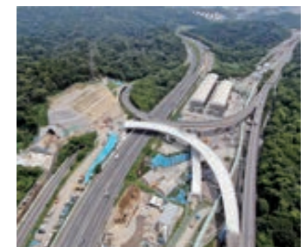
Construction around Kamaria JCT
