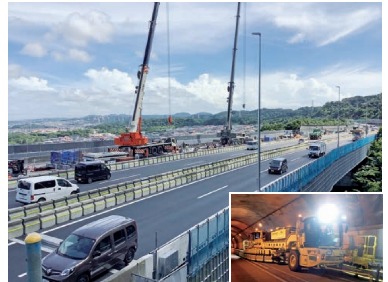
Deck slab replacement construction (Kamariya Daini Viaduct, Yokohama-Yokosuka Expressway)
